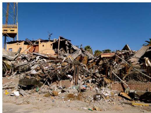
A building in Tripoli destroyed by a NATO strike.
